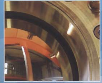
Segment in lowered position
